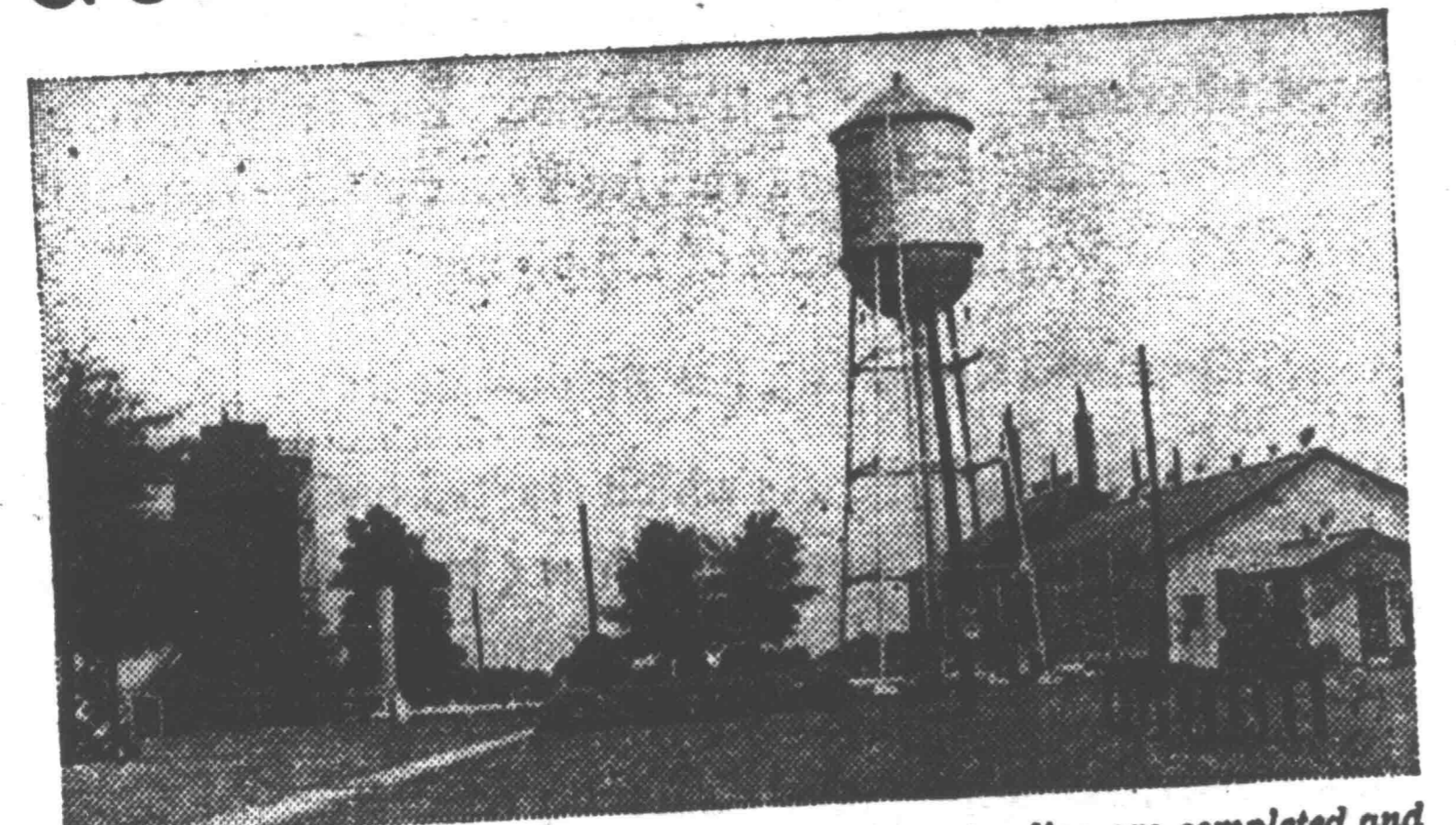
When new compressor stations on the Texas Gas pipe line are completed and landscaped they will look like this one on the Company's existing system.
